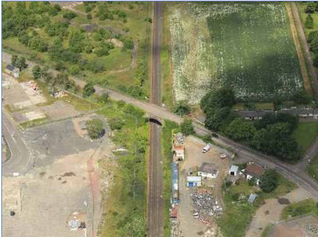
Aerial image of bridge site, looking north
