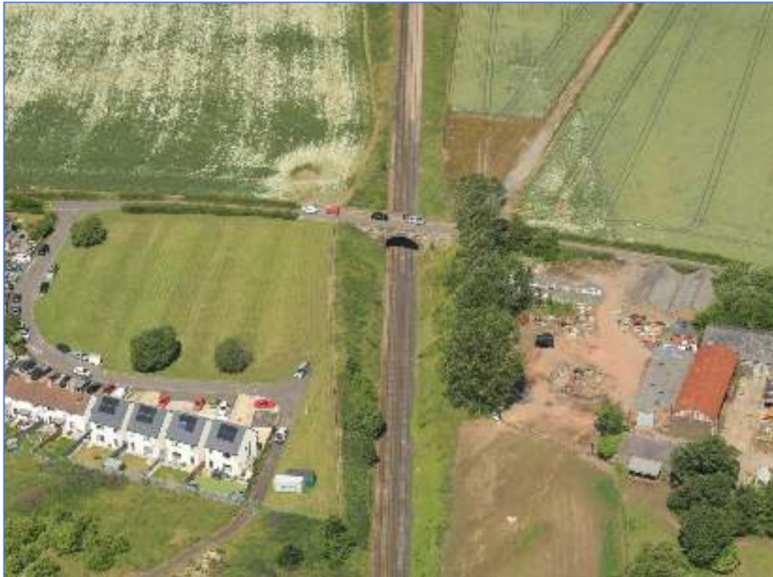
Aerial image of bridge site, looking north
